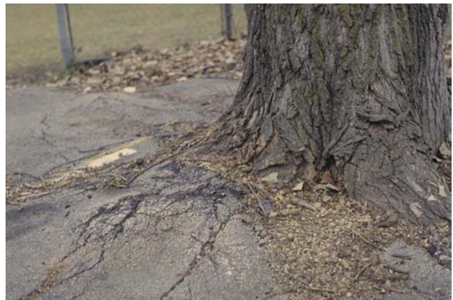
Addition of asphalt around base of tree
